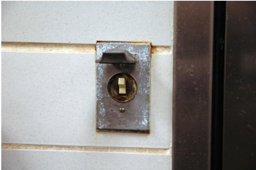
A light switch with residue build-up and grime. The switch could be contaminated with *Lm* by employees' hands during operation, and may not be cleaned during sanitation. When the light is turned on the next day, the hands could be re-contaminated.
